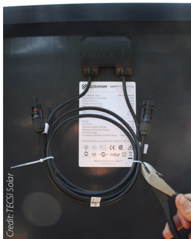
Figure 12. Removing standard factory installed wire ties
