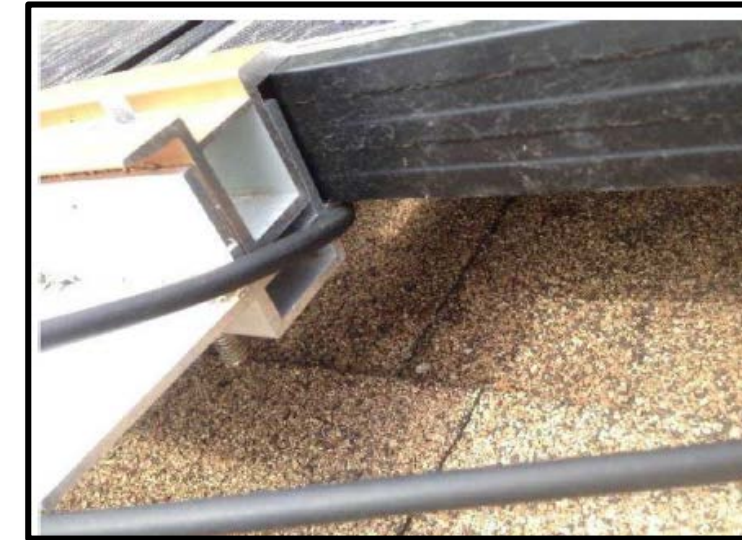
Pinched/Cut Wires
